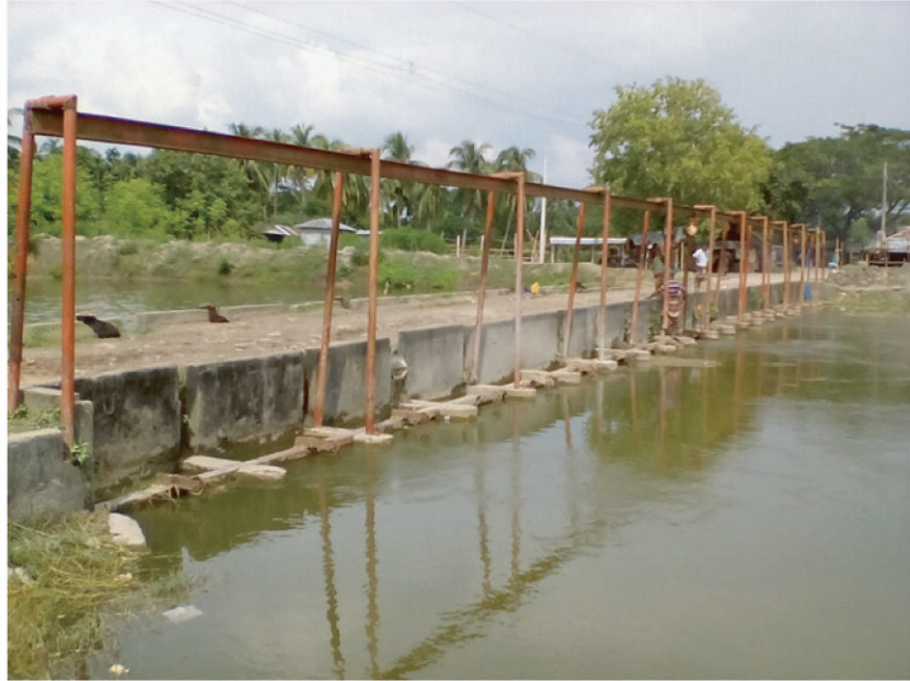
Bhabodah Sluice gate
